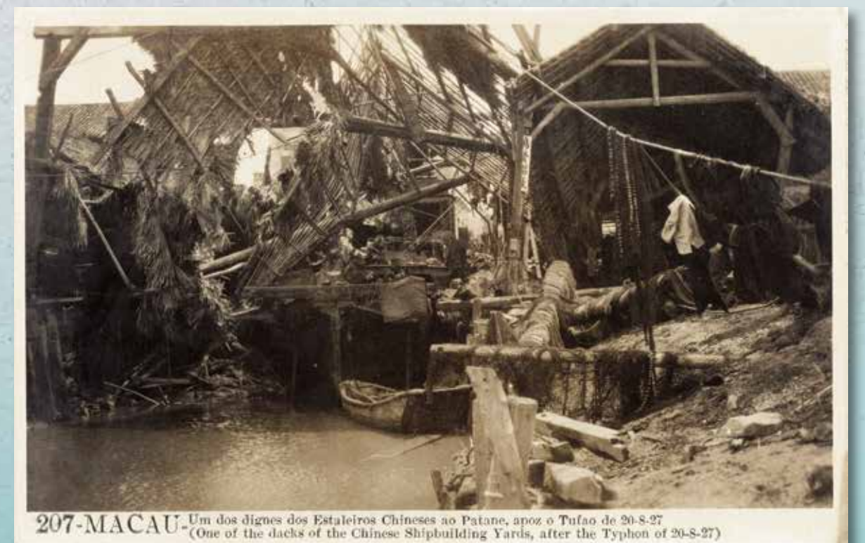
1927/08/20 颱風吹襲後的沙梨頭造船廠 Um dos estaleiros chineses no Patane após o tufão One of the Chinese shipbuilding yards in Patane after the typhoon 13.63 cm x 8.84 cm MO/AH/ICON/MTL/MO/531
